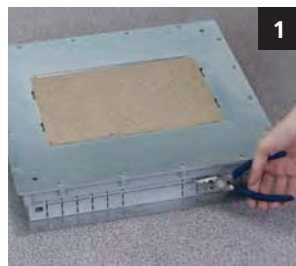
1 Cut the trunking inlets
