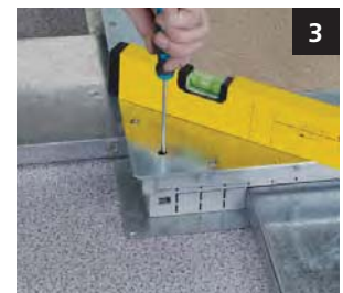
3 Level with the screws
