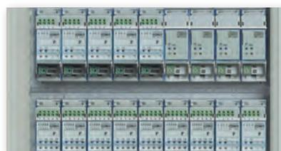
Area accessible to the installer with all the power supplies, actuators and other DIN devices (up to 288 modules) for the operation of the MyHOME system. The installation is completed with the white finishing panels.
