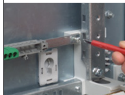
Fix the bar on the plastic supports integrated at the back of the cabinet
