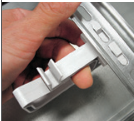
Fitting a guide ring for horizontal wiring
