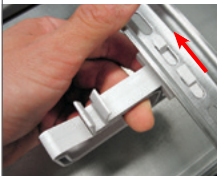
Fitting a guide ring for horizontal wiring
