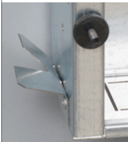
Pull up the masonry anchors
