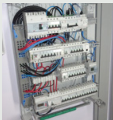
3-phase power supply to a row using the "three prong" type supply busbar
