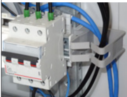
Holding vertical wiring in place
