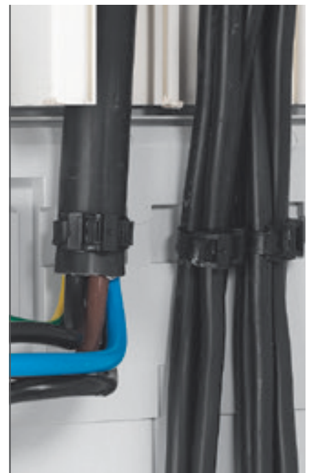
Anchoring the cables
