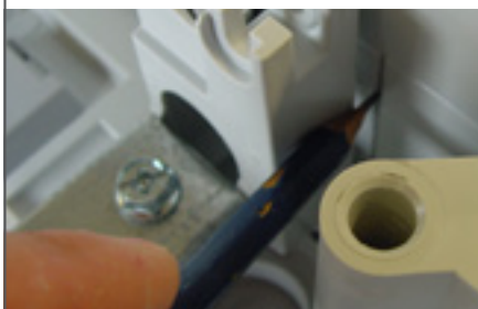
Use the terminal block supports as marking guides.
