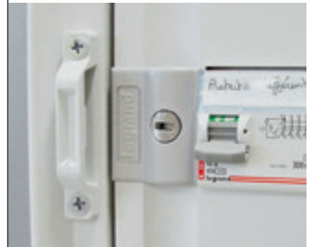
The door release is fitted on the opposite side to the hinges using 2 screws
