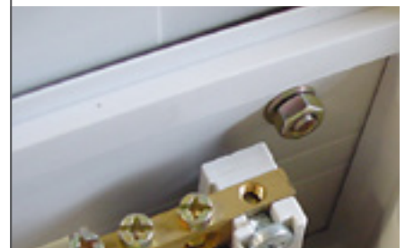
Place the 4 screws and 4 M6 nuts in position, but do not tighten them fully
