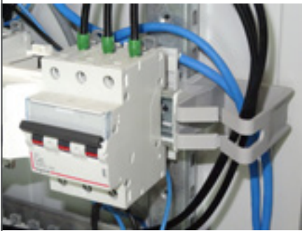
Holding vertical wiring in place
