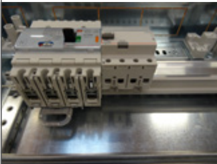
Installation of a modular product at the same level as the DPX 3 160
