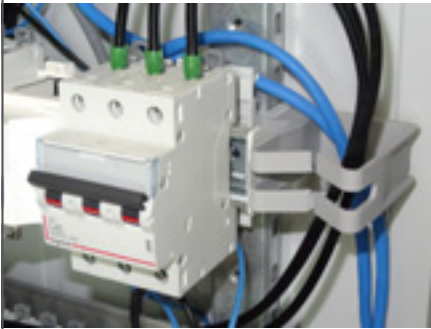
Holding vertical wiring in place
