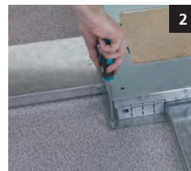
2 Insert the trunking and screw to the floor
