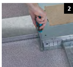
Insert the trunking and screw to the floor
